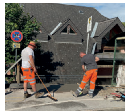
▲ Fundament E-Ladestation
