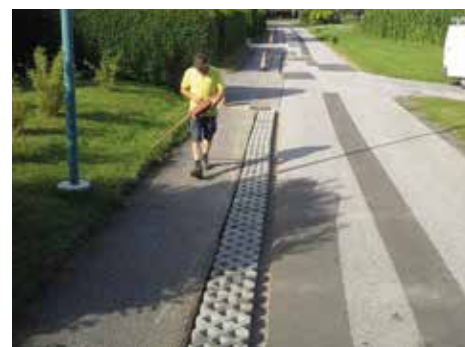
Rasengittersteine am Kremsweg in Walkersdorf
